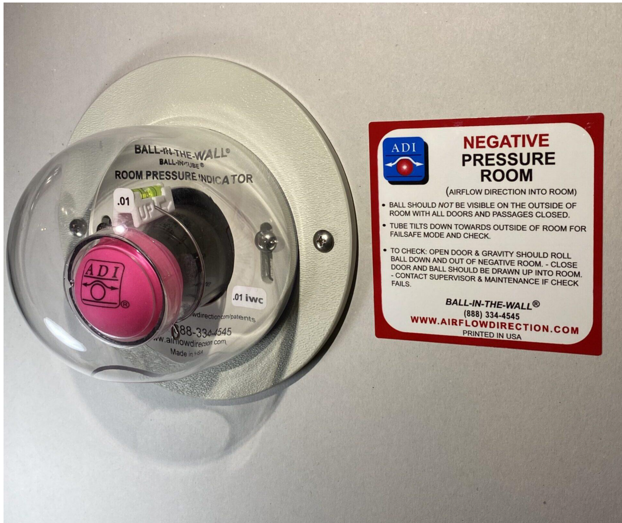
NEGATIVE BALL-IN-THE-WALL® SHOWN ALARMED AS VIEWED FROM OUTSIDE OF NEGATIVE ROOM. Note pressure setpoint label (0.01 iwc)
